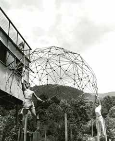
Dome being assembled
